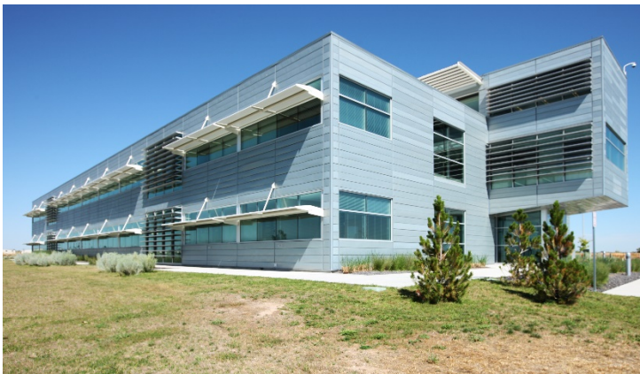
Center for Advanced Energy Studies, GSBS Architects Idaho Falls, Idaho Photo credit: Kevin Van Den Wymelenberg
